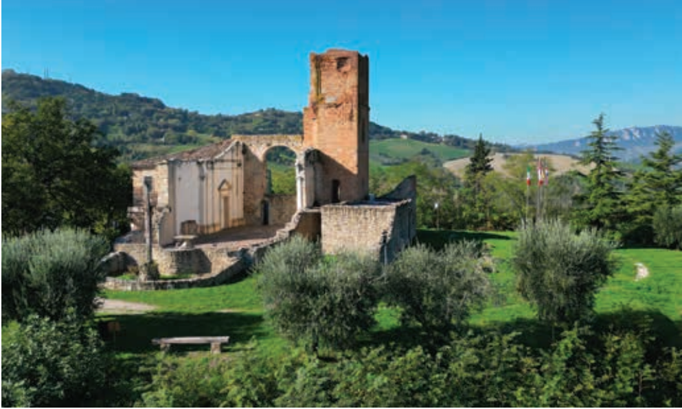
Trarivi, Ancient Peace Church and rectory, home to the Eastern Gothic Line Museum
